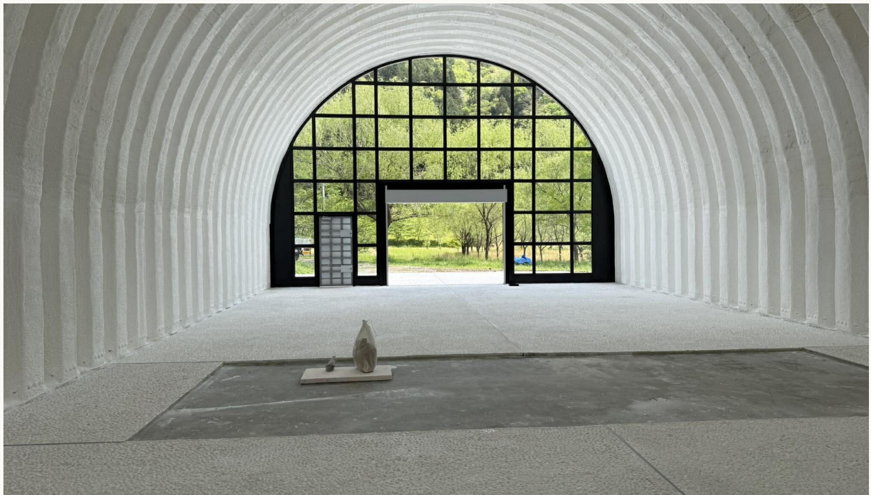
FIG. 9 Inside the vault — the white plaster ceiling in place, the lunette window framing the green hills. The floor and the interior walls remain in progress.
